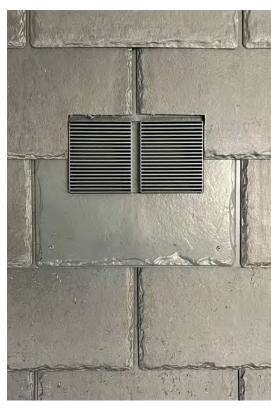
**Note:** The Liteslate tile vent is suitable for air or extraction ventilation, such as soil vents or air extraction, but is not suitable for heat extraction. Be aware that the tile vent is vacuum formed, so the finish and colour may slightly differ from the slates and other accessories.
